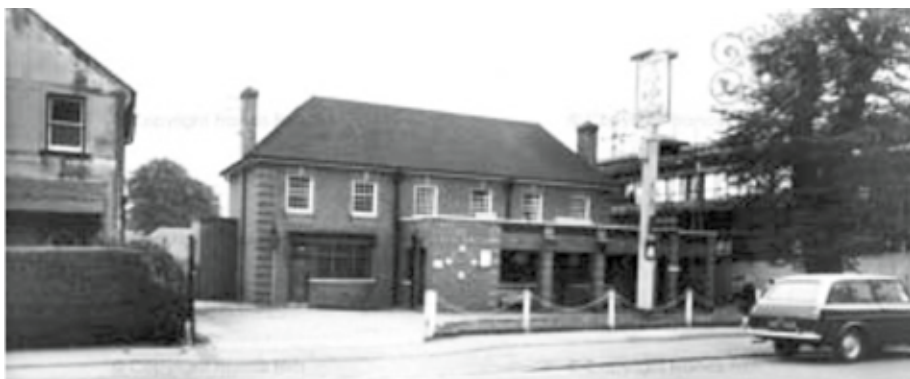
Photo of The Good Neighbour attributed to 1965 The Good Neighbour, built in 1956, became The Stag in 1983.
