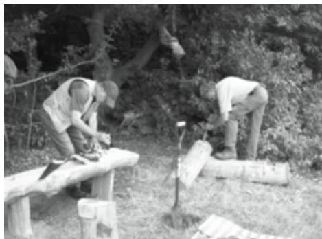
Installing a hand-made seat approx. 20 yrs ago
