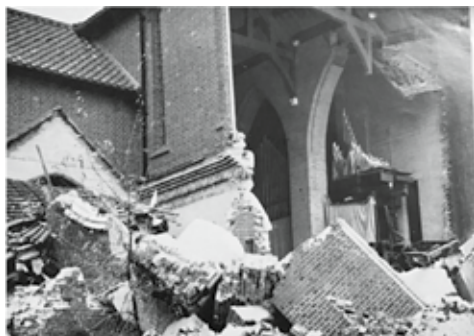
Detail of damage to St John the Divine from photo in Croydon Library Archives
