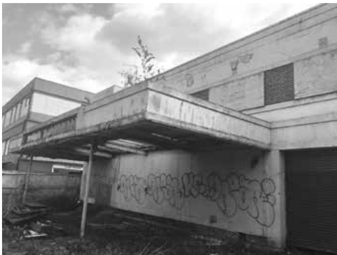
The once proud petrol station frontage.
