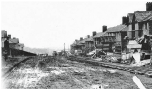
Top of Farley Road with Costain's narrow gauge railway bringing building materials up the hill to build Selsdon Garden Village
