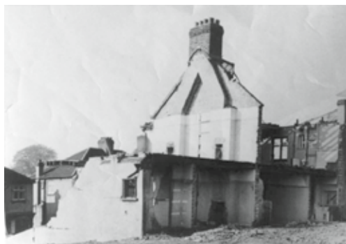
Photo of rear of Nos 41 / 42 Ingham Road
