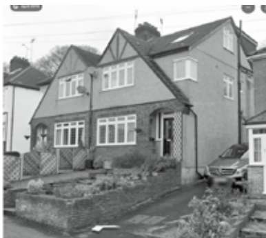
Nos 41 and 42 Repaired and reconstructed (from Google)
